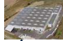
Holyshov Plant Czech Rep. 110,000 sqm Substructure production
