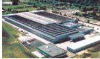
Ligny Plant France 175,000 sqm
